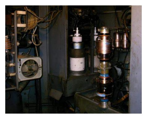
You are looking inside the back of a vintage BC-10B transmitter, in a small market station. The plate overload was tripping, taking the station off the air.
