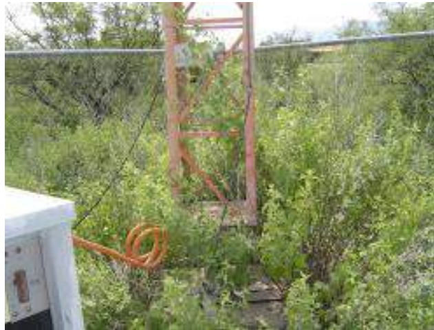
Eventually, when there is enough growth, it can even shunt power to ground
