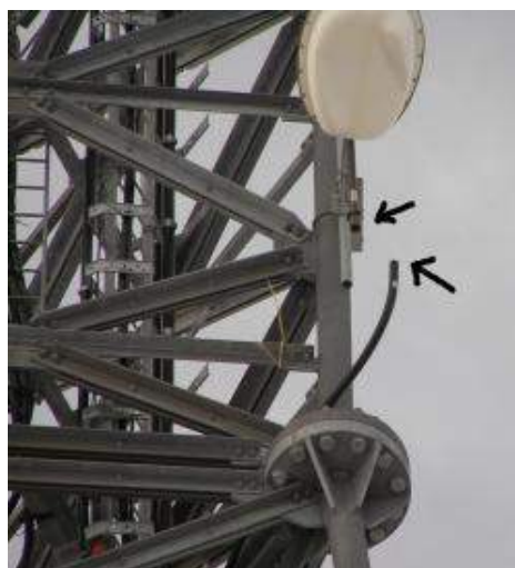
The line to this aux antenna was not continuous
