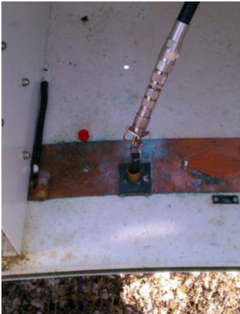
A chain of connectors bridges the gap
