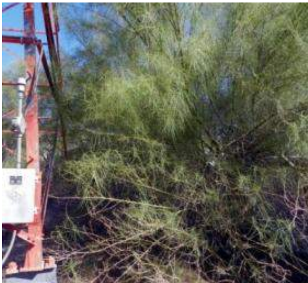
Even when there are no guy wires, out-of-control foliage can affect the radiated signal
