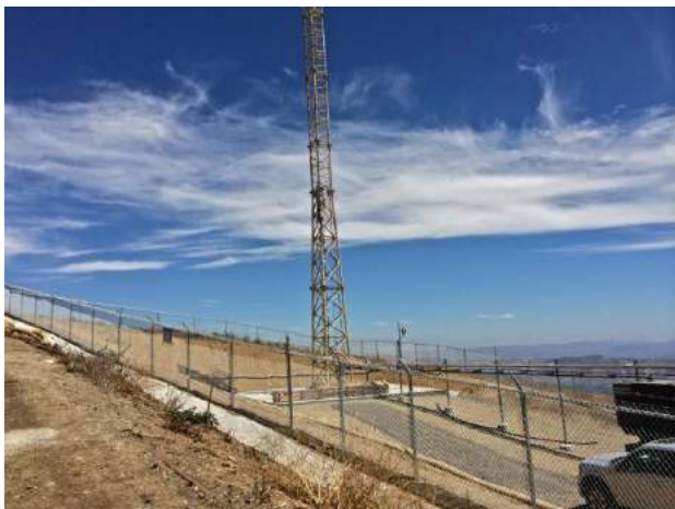
A site ready for RFR sign installation
