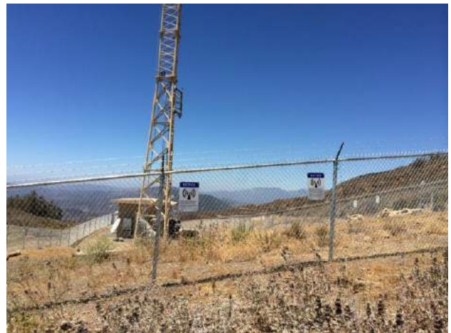
Two of the signs mounted (hopefully) for years to come
