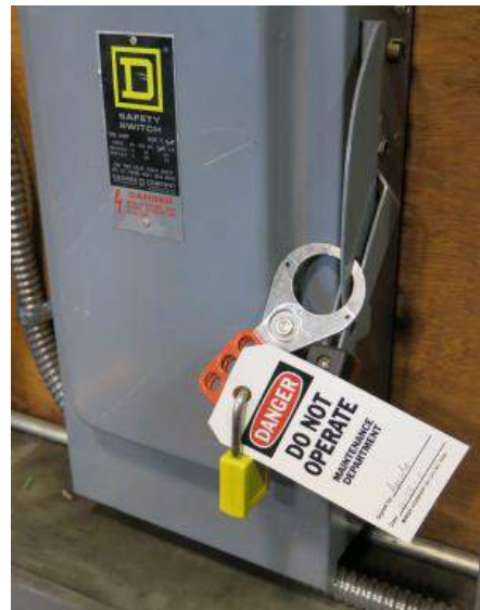
If you lock out a breaker, it is much less likely An unaware co-worker will try to turn it on.
