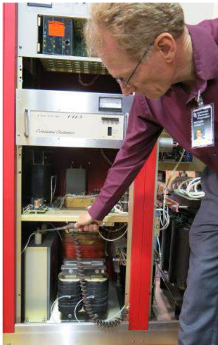
Proper use of the shorting stick can prevent unwanted surprises
