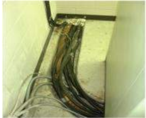
Foam coax entry points to keep critters out
