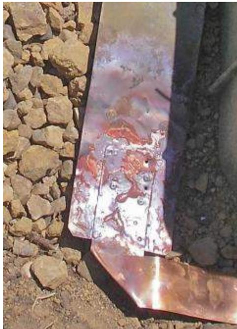
**Brazed joint after copper pop rivets were installed.
