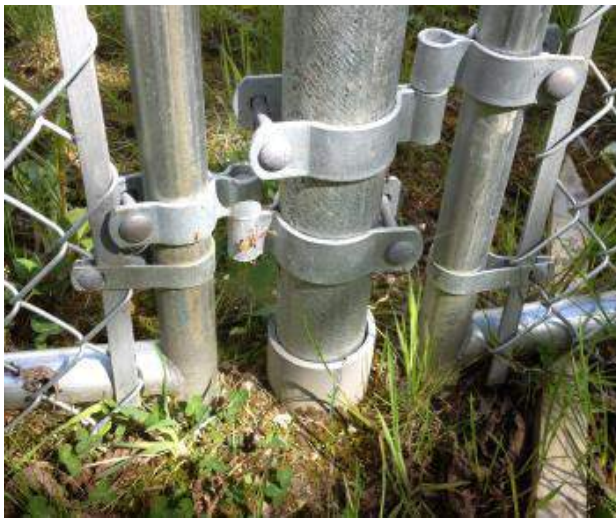
The fence poles fit nicely into pieces of 3-inch PVC conduit
