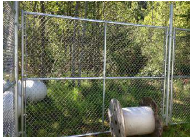
The sections hung easily on the hinge brackets
