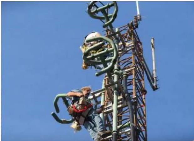
An ERI crew at work inspecting and replacing insulators
