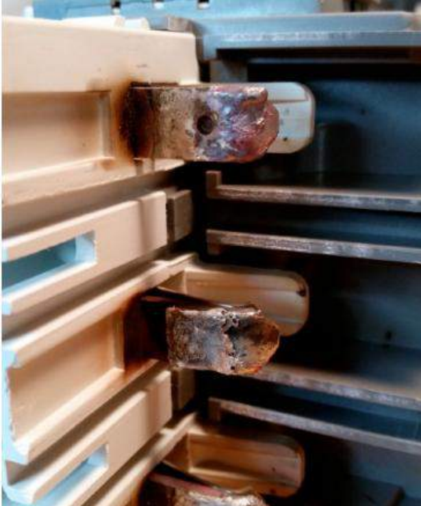
This connection exhibits the results of intermittent operation over some time
