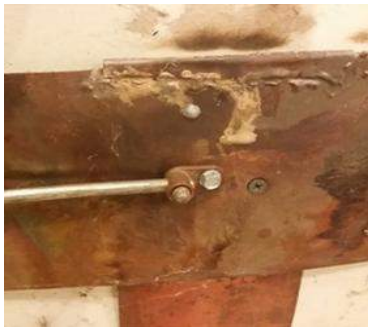
Sheet metal screws are not enough to ensure a solid ground
