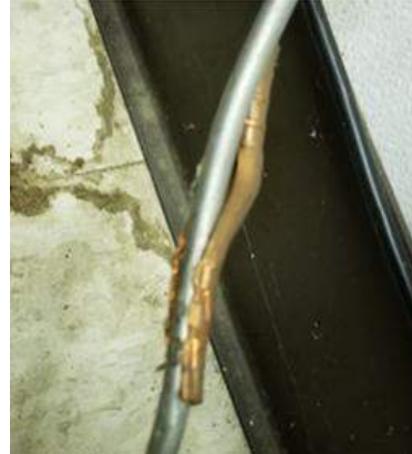
Well, it is crimped ... sort of ...
