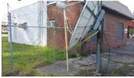
The strap runs down and under the lower edge of the dish and hooks near the dish mount hinge point. With the winch, I put enough pressure on the dish to be able to easily loosen the elevation hardware and then raise the dish using the winch.
