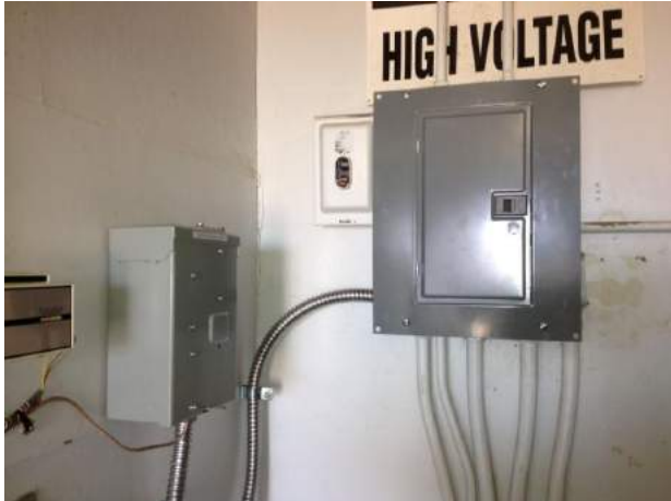
After the enclosure was installed the wiring looked much cleaner
