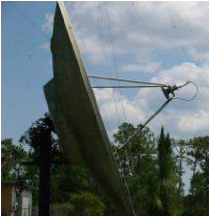
The feed horn is askew in relation to the dish
