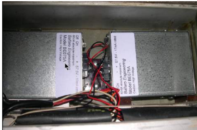
Two BE675A modules installed in an N-C 120B to replace the two B batteries.
