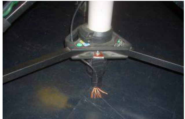
The solder wick provides contact with the floor
