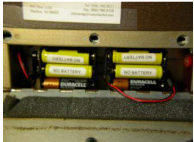
Compartment with two, 6-cell, battery packs.
