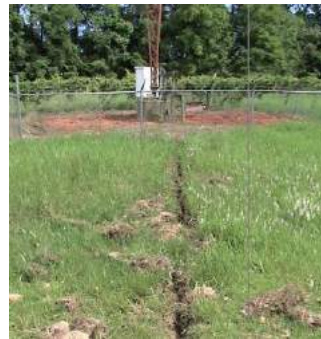
No one wants to see something like this, where the copper has left the ground
