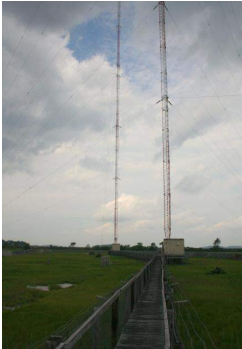
The elevated tower bases and walkways keep the tidal waters well below the towers
