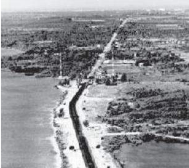
Looking West along the Davis Causeway
