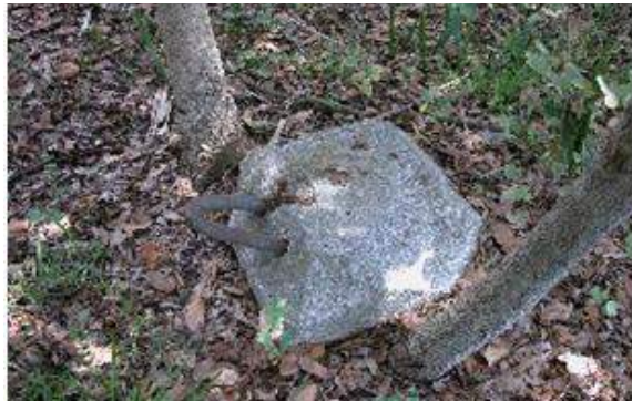
The East Guy Anchor from the North Tower
