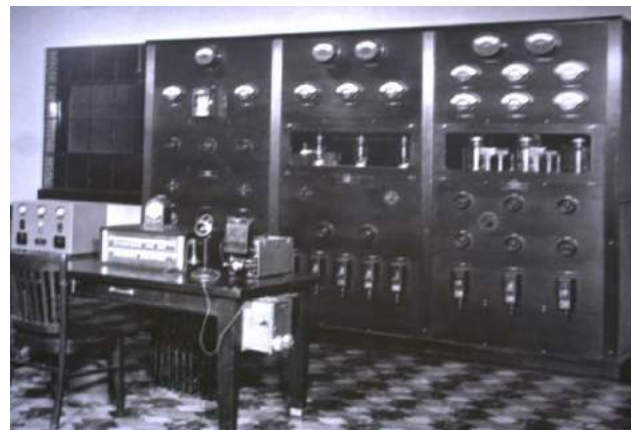
As the station grew, a larger transmitter helped
