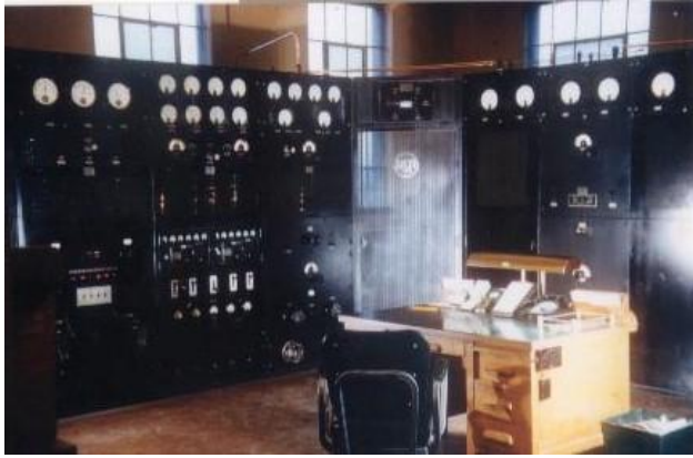
The RCA 50B transmitter was upgraded and kept the station on the air until 1959.
