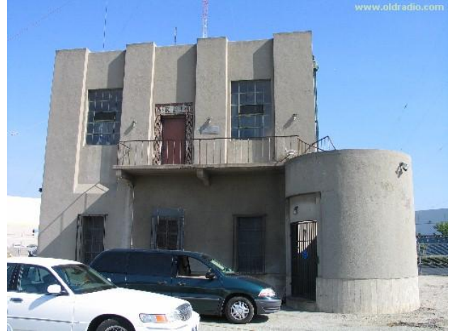
The KFI transmitter building
