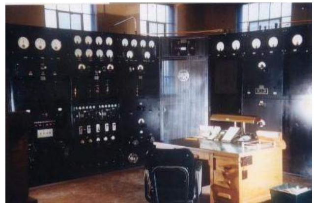
The RCA 50B transmitter was upgraded and kept the station on the air until 1959.
