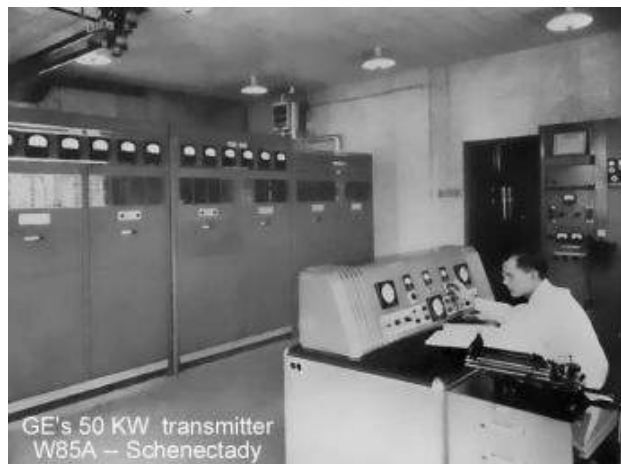
GE's 50 kW FM transmitter used in early WGY-FM operations
