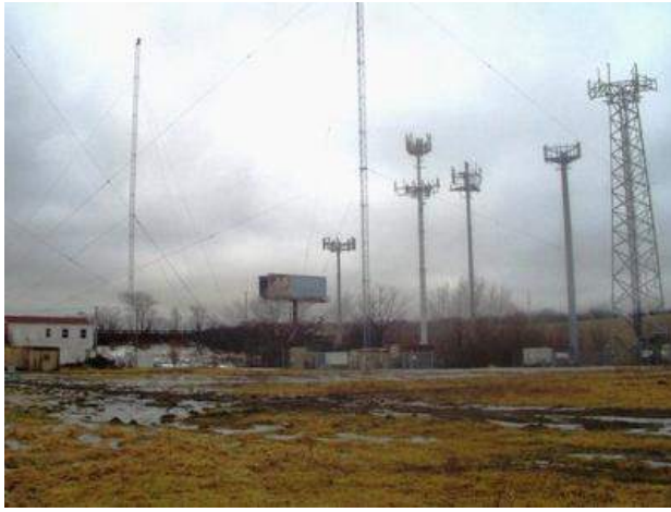
This AM directional site has several detuned cell towers in close proximity
