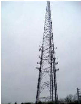
On this particular self-supporter the actual AM antenna is an 8-wire skirt.
