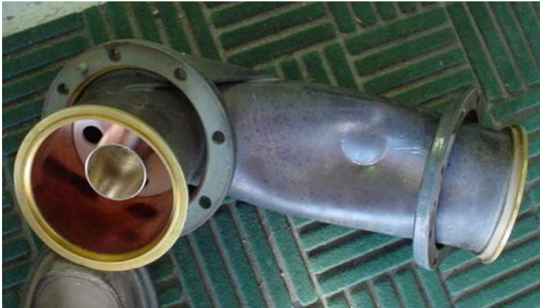
This elbow was damaged when a crew working for a co-located station dropped a 10-foot piece of conduit on it – and was then ready to leave the site without telling anyone. Photos: Gary Peterson
