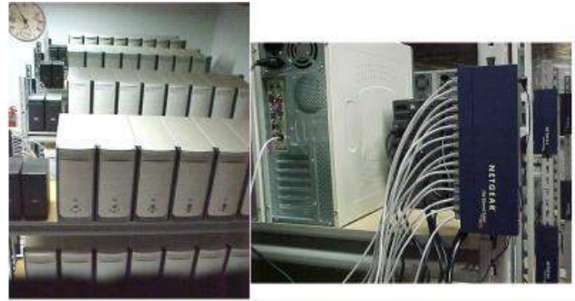
The cluster computer in these photos has been used to design 50 kW upgrades for directional AM stations in Detroit, Baltimore, Boston and Chicago.
