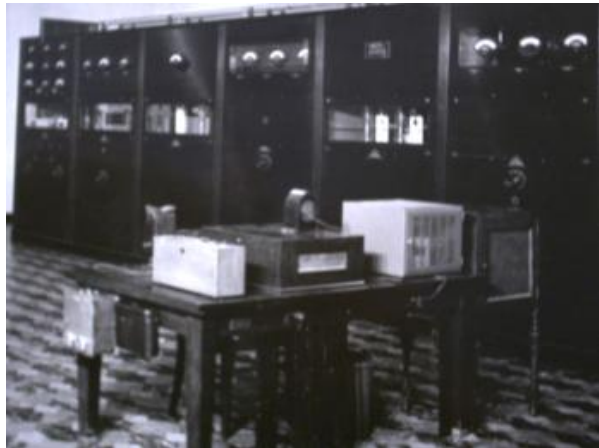
A Western Electric 7A transmitter brought KSL to the top power level of 50 kW.
