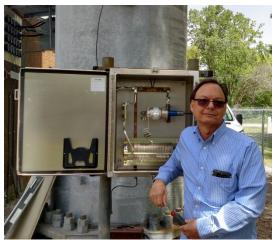
Any detuning network on a skirt must be assessed and adjusted if tower work causes changes
