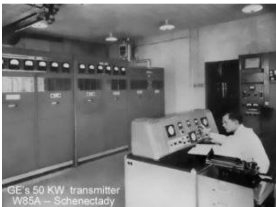
GE's 50 kW FM transmitter was used in early WGY-FM operations
