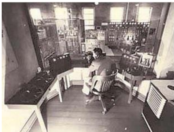
A transmitter viewed through the CR window
