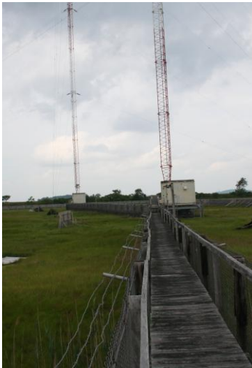
The elevated tower bases and walkways keep the tidal waters well below the tower bases
