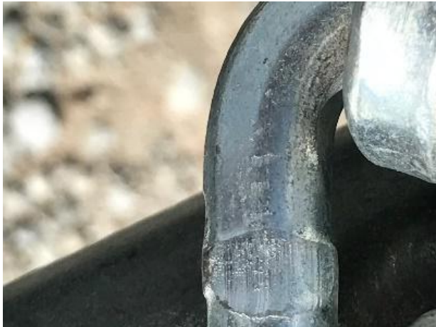
Notice the tool marks on the chain
