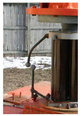
First, they limit the static charge build up on the tower by furnishing an easily ionized path for
