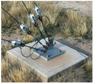
A guy anchor encased in cement with turnbuckles and insulators
