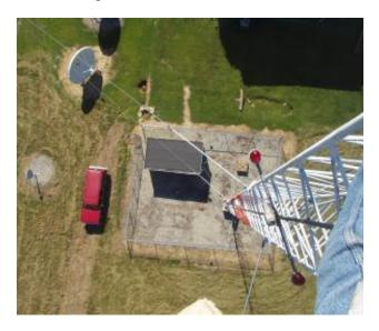
A "bird's eye view" will sometimes expose things in the field, or at the anchors, that just will not be seen from the ground – or are just too easy to miss while on the ground. For example, from the top, it is pretty easy to see if a tower is kinked, twisted, or otherwise out of plumb.
