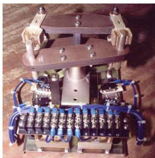
The contactors at tower bases are usually the most heavily stressed physically, especially the solenoids and finger stock.
