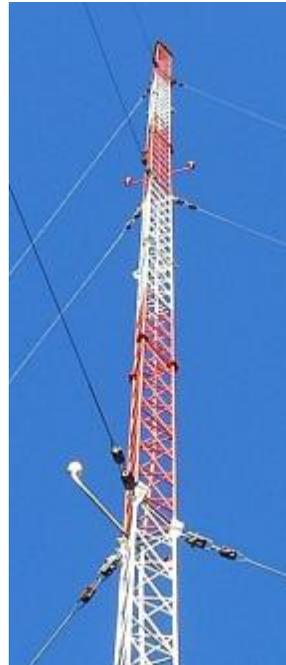
KDON's towers stood 198 feet above the base insulators, four feet off the ground. Each tower, then, was 202 feet, six inches high. And I had to conquer every inch on both towers.
