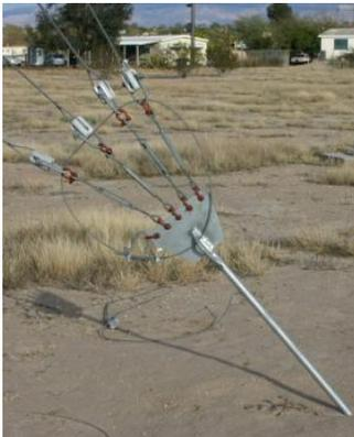
As a real world example, notice this guy anchor. There are some things that are done properly, including the insulators and the loop to prevent tower vibrations from affecting the turnbuckles.
