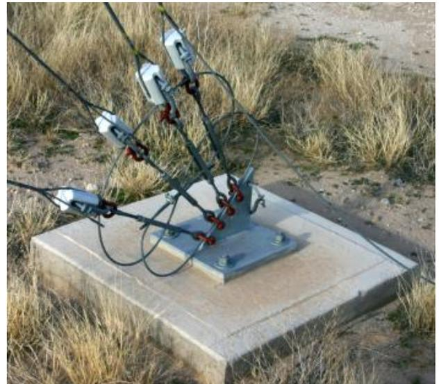
**A guy anchor encased in cement with turnbuckles and insulators**
