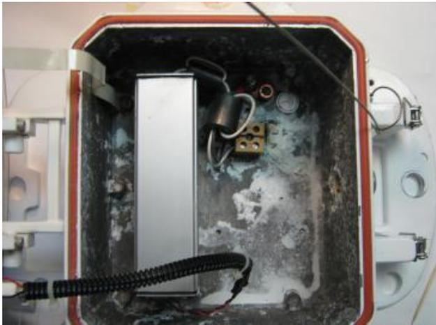
After we dried it out and, as a test, temporarily bypassed the power connection strip which was severely corroded, the light came on immediately with no indication of any malfunction.
