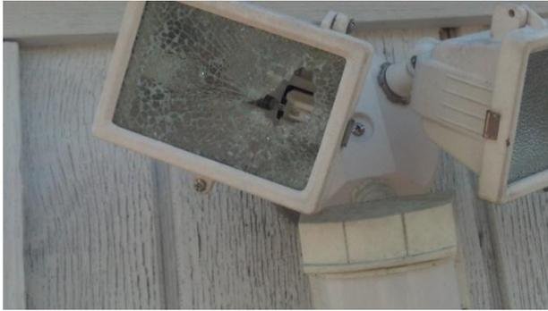
In most cases, the fixture and bulbs were physically broken. In a few cases the vandals simply unscrewed bulbs or, in even fewer cases, moved the light fixture away from the area in which they would be “working.”
