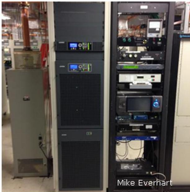
The Flexiva FAX20 is narrower than a rack
