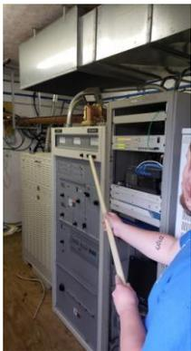
Here is a photo of Hartman turning a tube transmitter back on with a wooden broom handle after cleaning snow out of the transmitter and drying everything off ("long story," he says). He says "This particular 20 kW transmitter runs at about 8500 Vols with 2.5 Amps across the plate. If it's unhappy, it goes BANG very loudly and you don't want to be right in front of it at the time."
