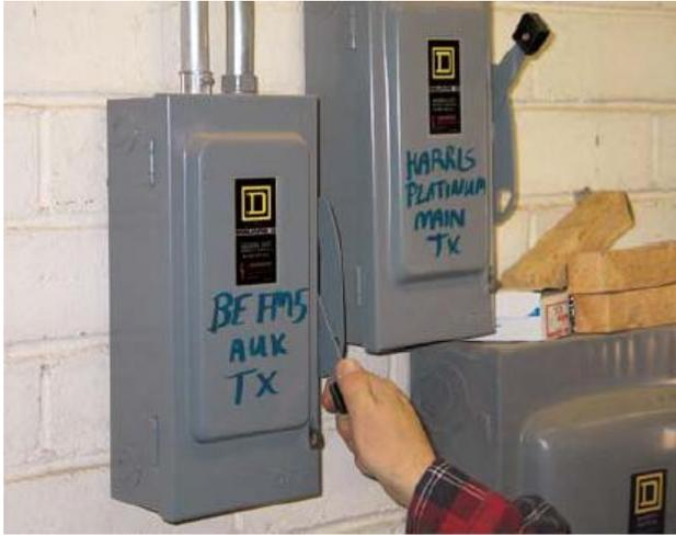
**Clear marking prevents mistaking which breaker feeds which transmitter**
