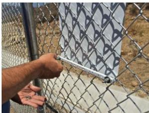
Each hole was filled with a 2-inch zinc-plated carriage bolt with a fender washer for strain relief, and a washer nut, lock washer, and a second nut
