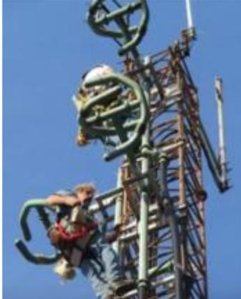
This side-mounted antenna is an example where we reported the insulators had started to deteriorate due to solar exposure after 25 years. You could see where they were leaking and where they were layered.
