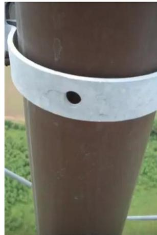
Here is a shot of a transmission line that actually runs through the aperture of the bays of an active side-mount FM antenna. You can see it is missing one of the little insulating buttons that keeps the rigid line outer conductor from touching that metal hanger.
