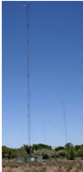
Using folded unipoles In a three-tower directional
