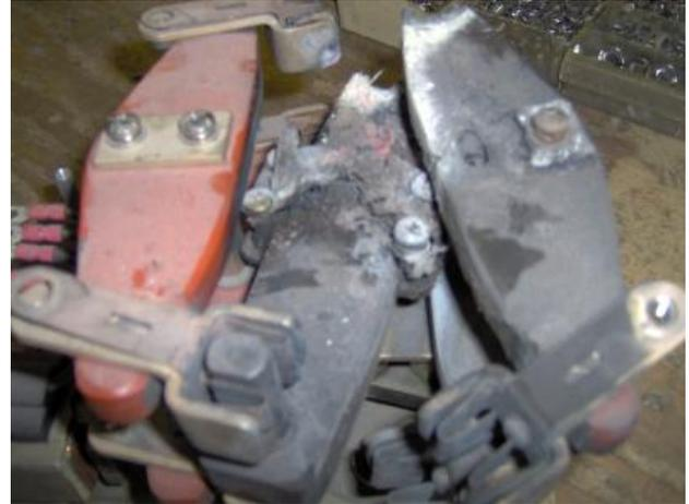
**Moisture caused this contactor to burn**
