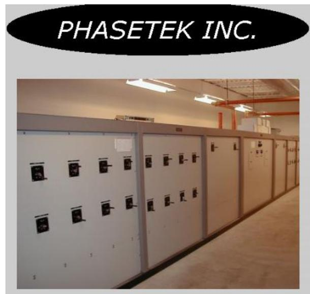
Ensure you have a complete parts list, understand what currents are present in the various branches of the system, and periodically check the components under load during maintenance visits. (An infrared thermometer is helpful in watching for unusual hot spots.)
