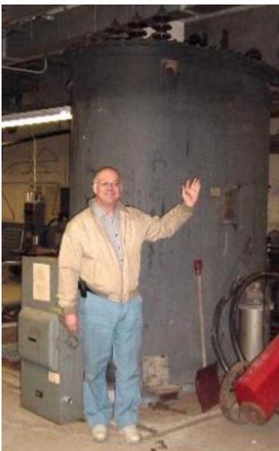
Each modulation transformer (left) weighed 35,700 pounds, including 725 gallons of oil, and was about 10 feet tall.
